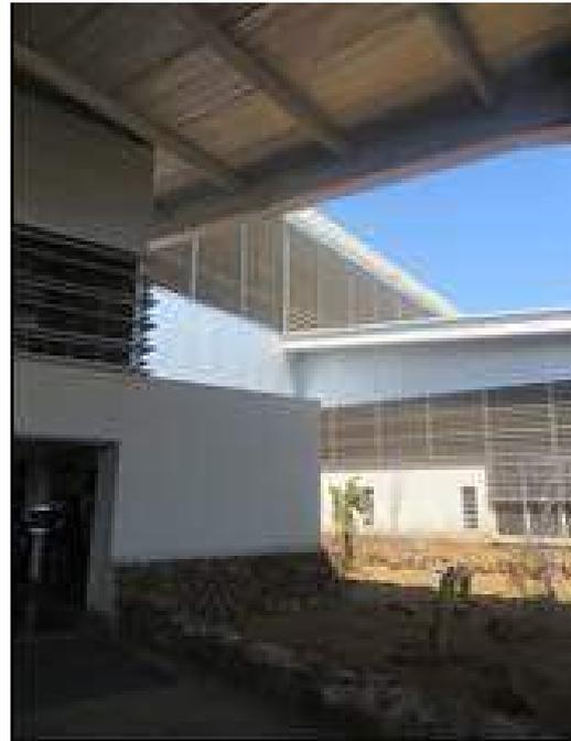
Figure 15. Openings with mosquito screening, without glass.
