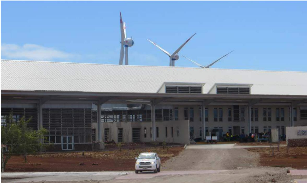
Figure 9. Airport passenger terminal showing the reflective white roof and the southern façade in total shade. The wind turbines to the north of the terminal provide part of the electricity demand.
