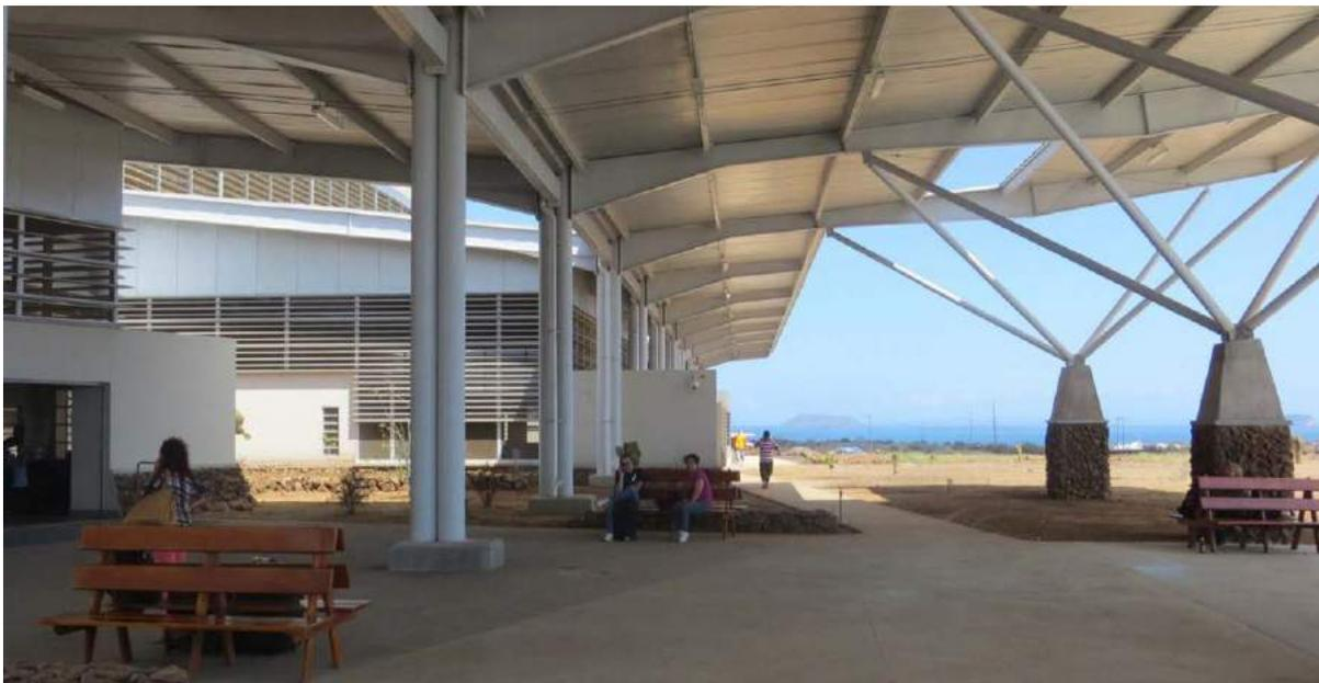
Figure 11. Shading of outdoor circulation spaces and building facades. Louvres on the east façade and white painted walls also reduce solar gains.
