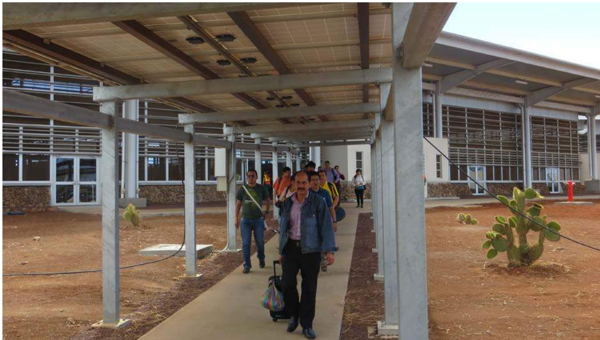
Figure 16. Two walkways, with photovoltaic roofs, provide 25 % of the electrical energy demand, as well as shade and rain protection for the path between parked aircraft and the terminal building.
